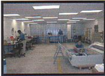
UL508A and UL913 certified electrical shop
